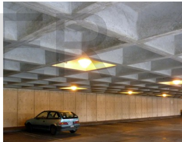
Fig 1: Typical waffle slab floor
